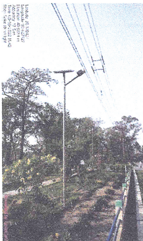
Figure 5: 30-Watt Solar Street Light Installed in the Campus
